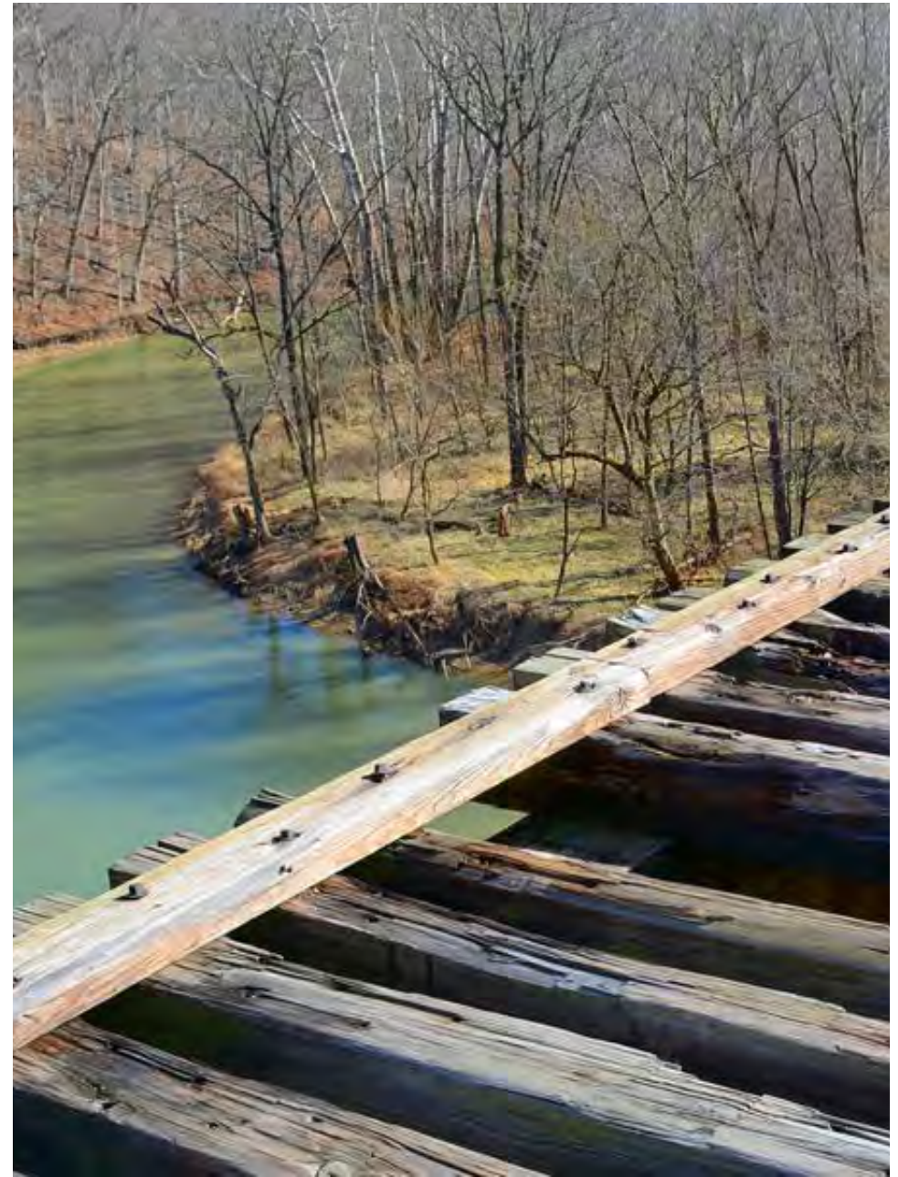
The Monon High Bridge spanning Deer Creek (image source: Pharos Tribune)
